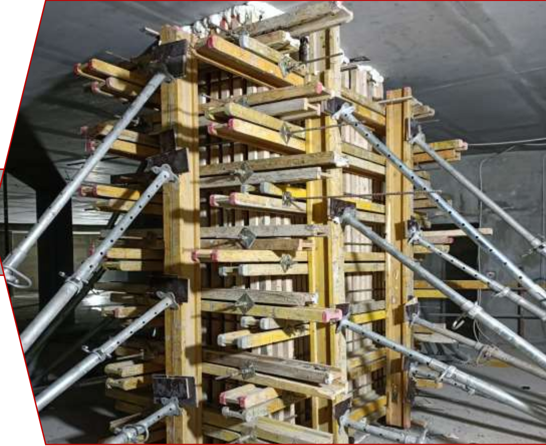
Shuttering works for column.
