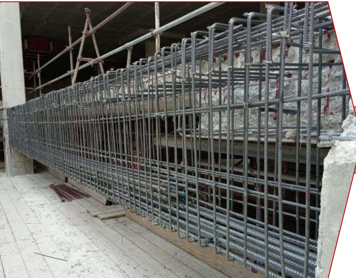
Beam Jacketing Reinforcement.
