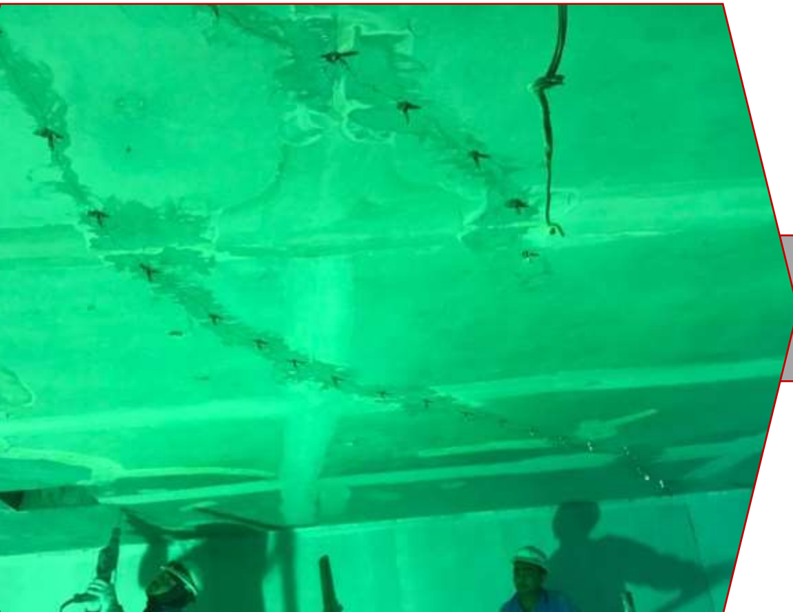
Cracks Injection.
