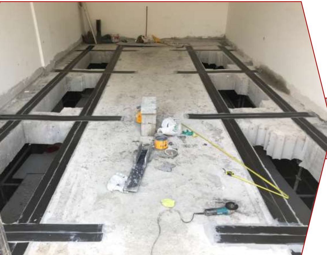
CFRP strips slab strengthening.
