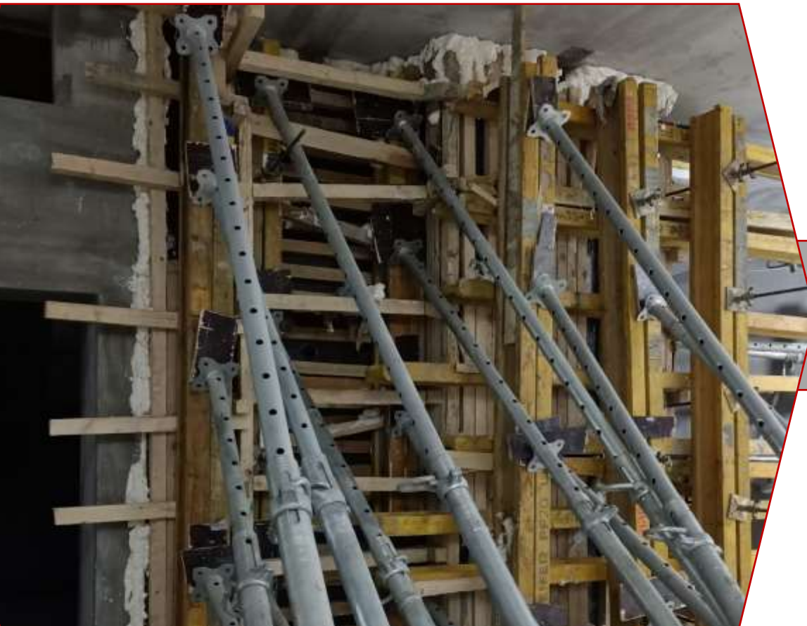
Shuttering works for R.C. wall.
