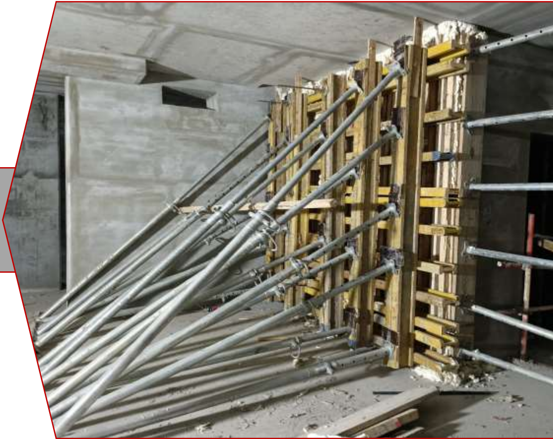
Shuttering works for R.C. wall.
