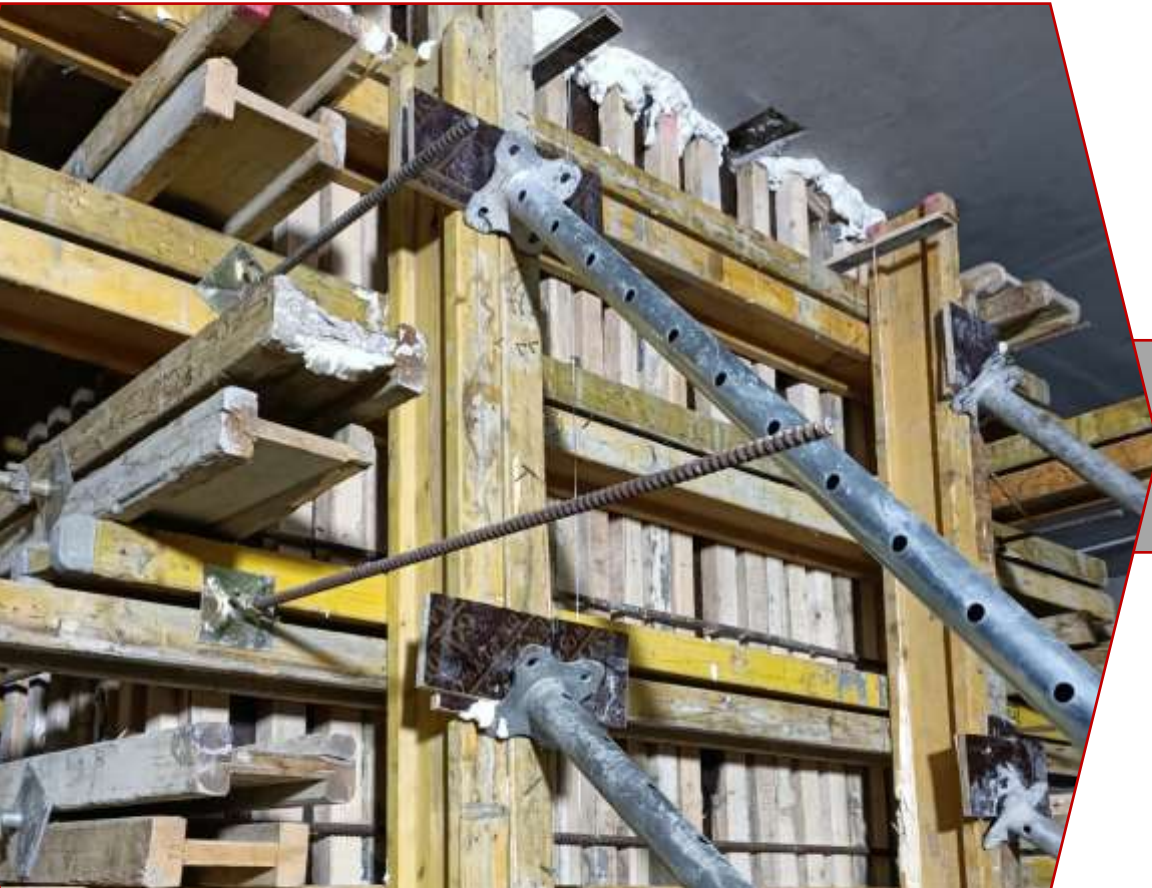
Shuttering works details for column.
