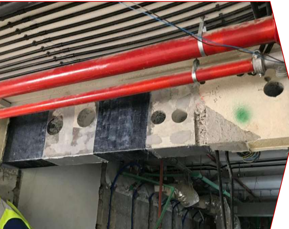
CFRP wrapping beam strengthening.
