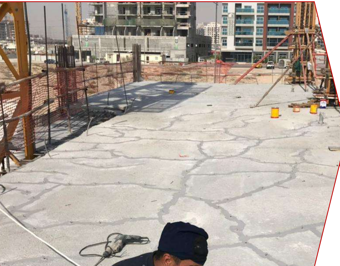
Cracks Injection.
