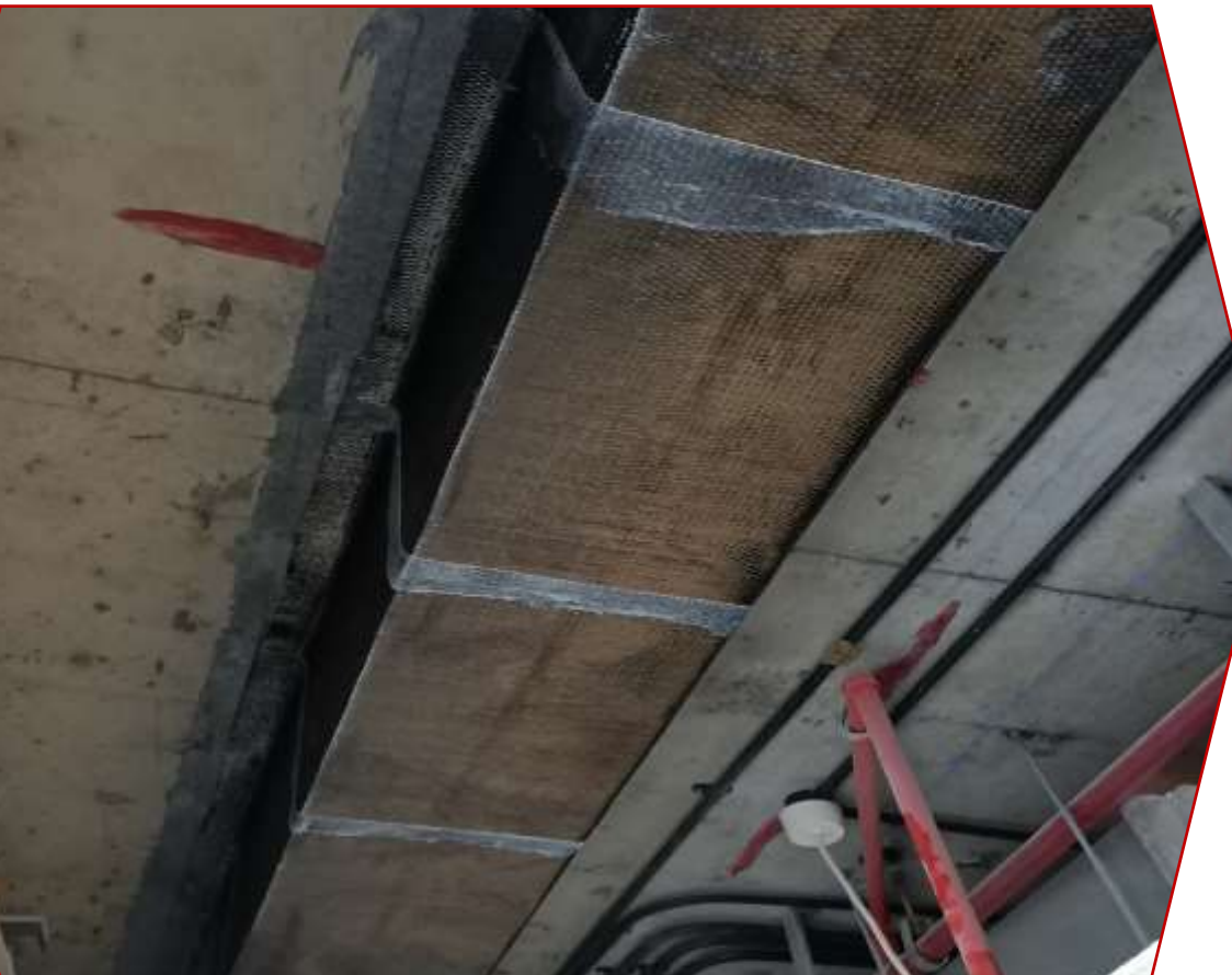
CFRP wrapping beam strengthening.
