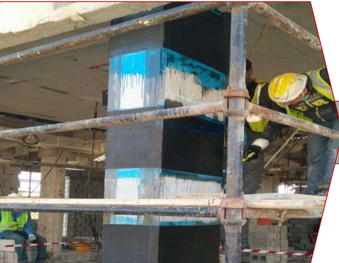
CFRP wrapping column strengthening.
