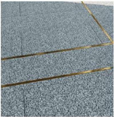
P06 - BRASS AND BRONZE STRIP - COLOR-GOLD - FINISH-POLISHED - CUSTOM SIZEX30MM THK.
