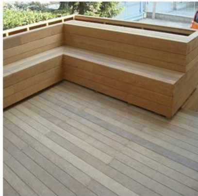
W03 - WPC TIMBER CLADDING - COLOR-BROWN - FINISH-NATURAL OAK - 100MM WIDE PLANKS X 20MM THK.
