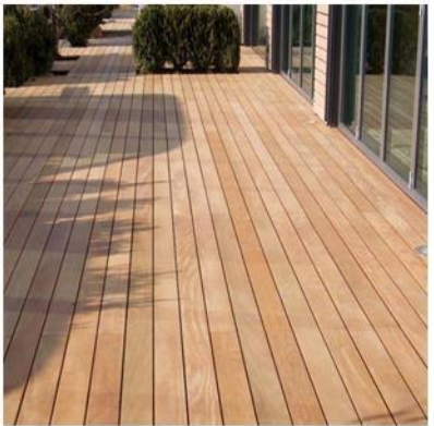
P11 - WPC TIMBER DECK - COLOR-BROWN - FINISH-NATURAL OAK - 100MM WIDE PLANKSX20MM THK.
