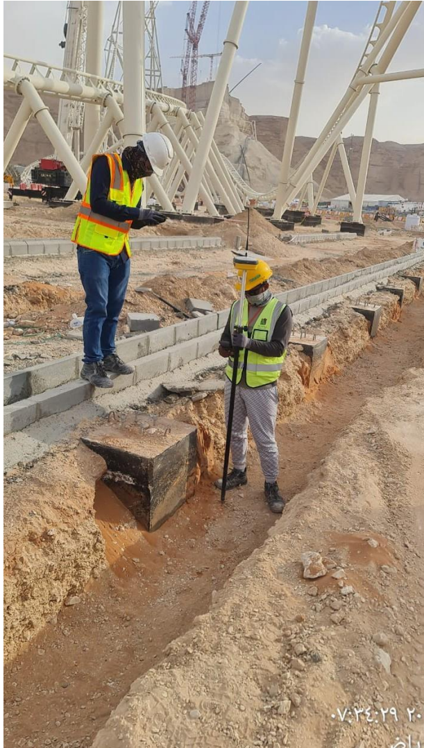
EXCAVATION AND SETTING OUT
