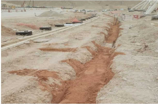
BACKFILLING
