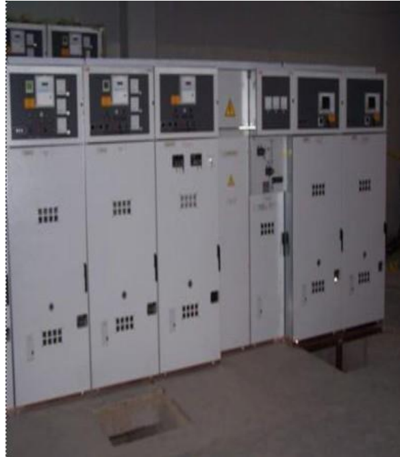
Replaced with ABB Unimix MV Switchgear
