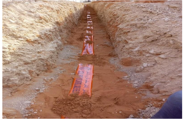
WARNING TAPE INSTALLATION
