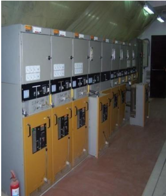
Old MV Switchgear
