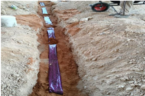
WARNING TAPE INSTALLATION
