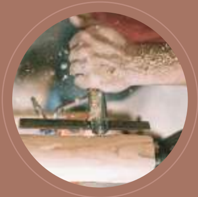
Fitted Joinery & Mill Works
